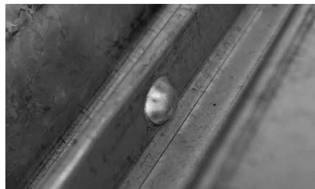
Figure 1.14.3: BUTTON PUNCH SIDE LAPS
