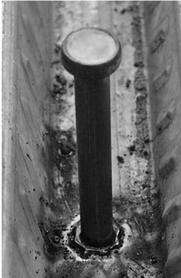
Figure 1.13.9: HEADED STUD ANCHOR
