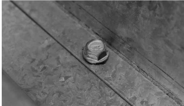
Figure 1.14.3: SIDE SEAM SELF-DRILLING SCREW (Nestable Sidelap)
