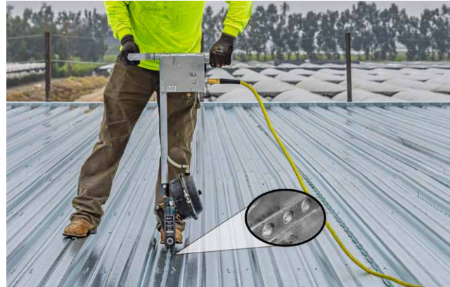
Figure 1.14.1: PNEUMATIC TOOL INSTALLING TRIPLE FLOOR CONNECTION
