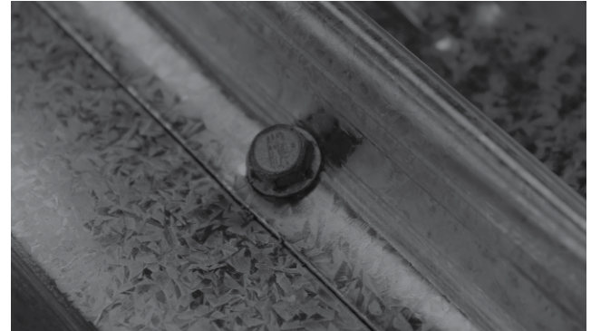
Figure 1.14.5: SIDE SEAM SELF-DRILLING SCREW (Screwable Sidelap)
