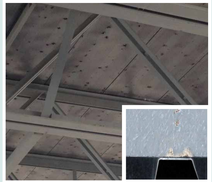
Exposed Welded Cell Deck - Unfinished
